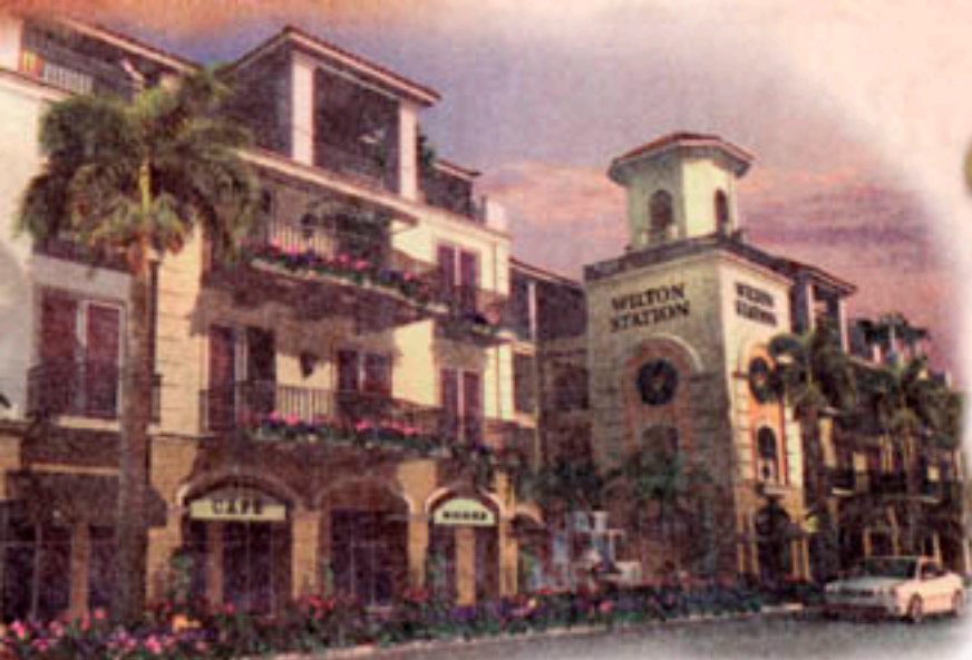
Wilton Station's signature clock tower is expected to become a landmark, reflecting the elegance of this mixed use urban village.
